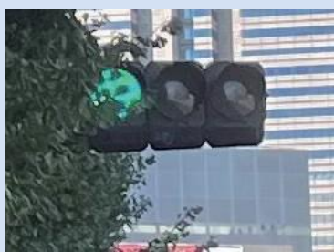
Lowered stoplight visibility
