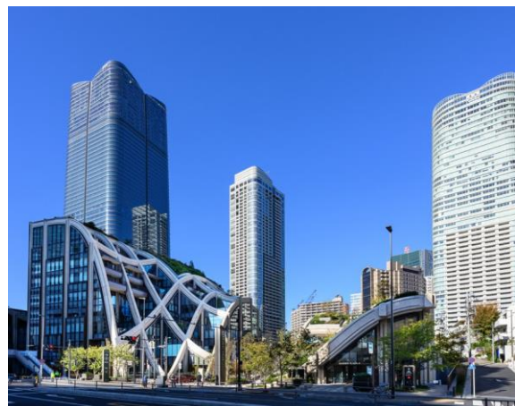
Green spaces leveraging local topography and greenery on low rooftops (Azabudai Hills)
