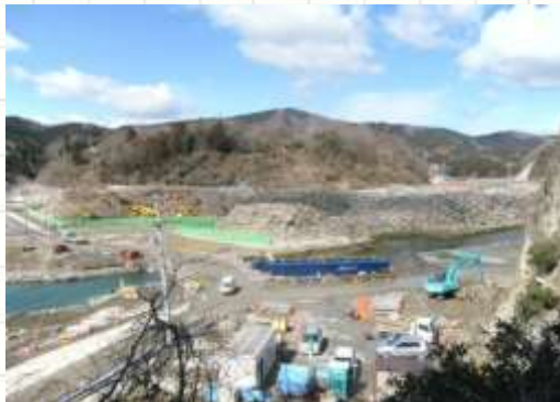
Waste from Great East Japan Earthquake (Onagawa town temporary yard)
