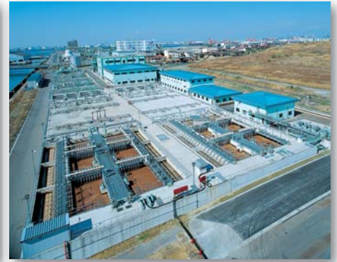
Wastewater Treatment Plant
