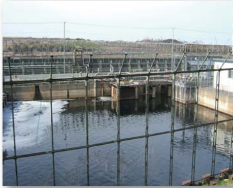
Receiving Reservoir (Pump well)
