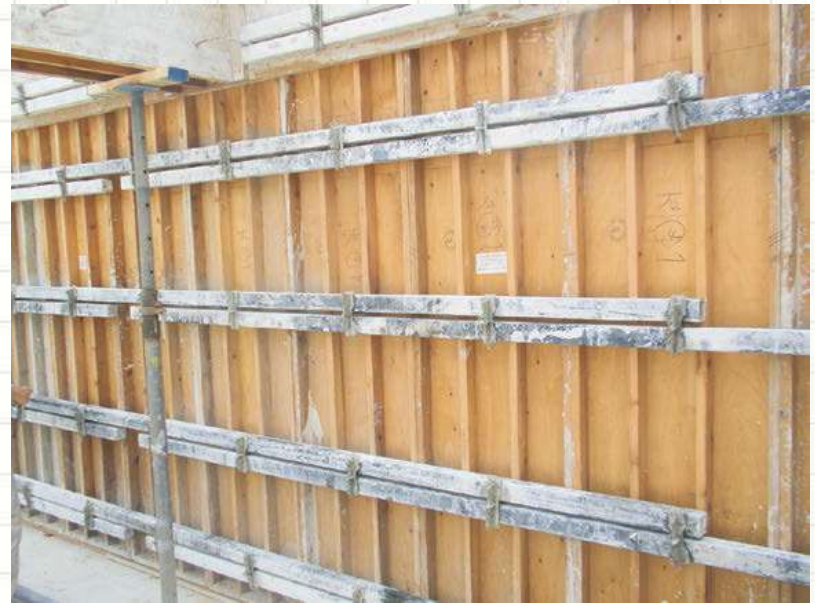
Concrete Forms using Domestic Lumber
