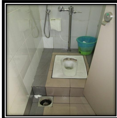
BROKEN TOILET BOWL NO GULLY TRAP COVER
