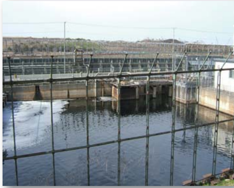
Receiving Reservoir (Pump well)
