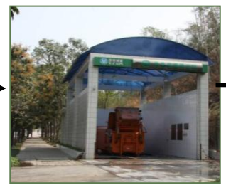
5 cum container to be placed at designated modified Dhalaos
