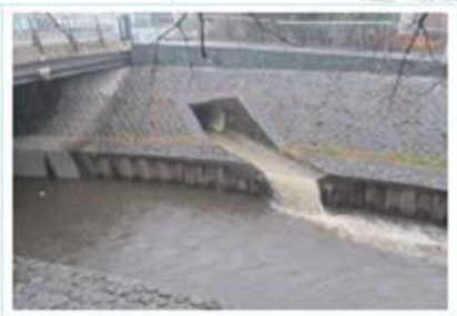
Discharge from sewer outlet
