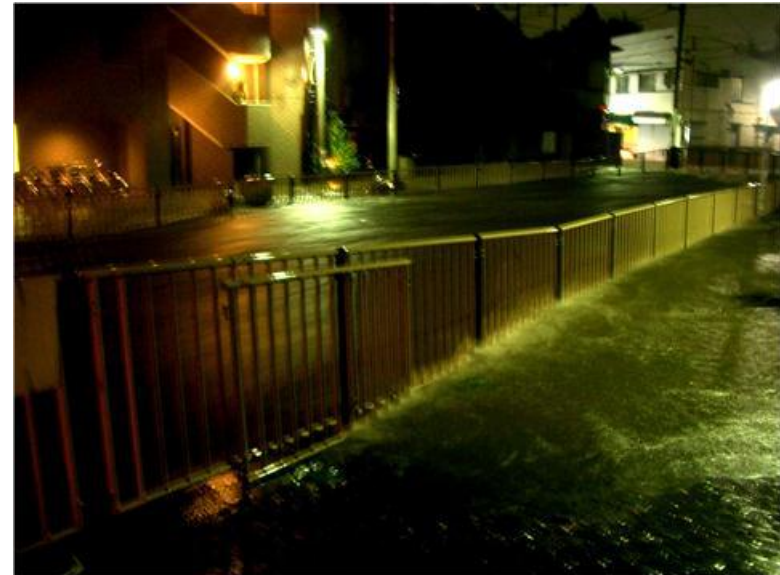
Torrential rains hit the metropolitan area in September 4, 2005 Josui Bridge over the Kanda River (1-chome Honan, Sugunami Ward)
