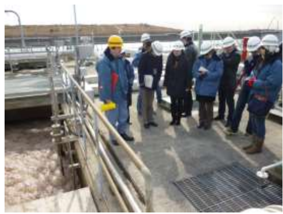
Waste water treatment plant at FDS
