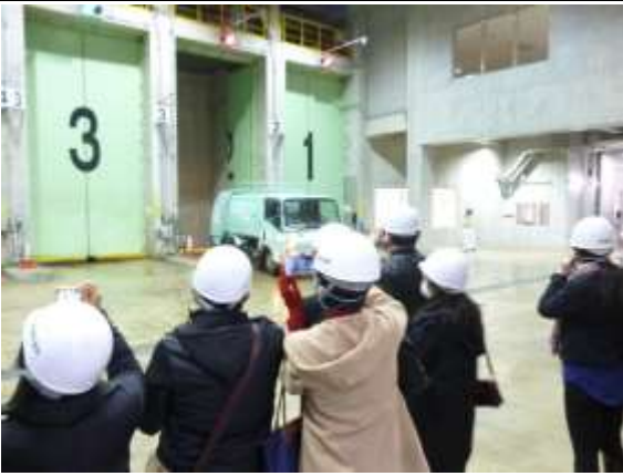
Incineration plant / Clean Center Fujimi
