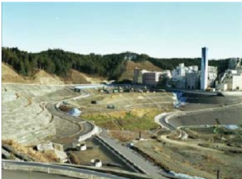
Futatsuzuka Final Disposal Site
