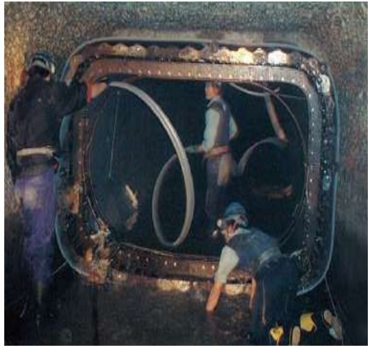
A sewage pipe being rebuilt
