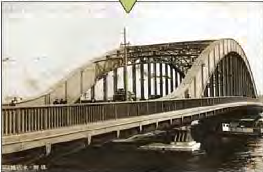
Eitai Bridge after Recovery Project
