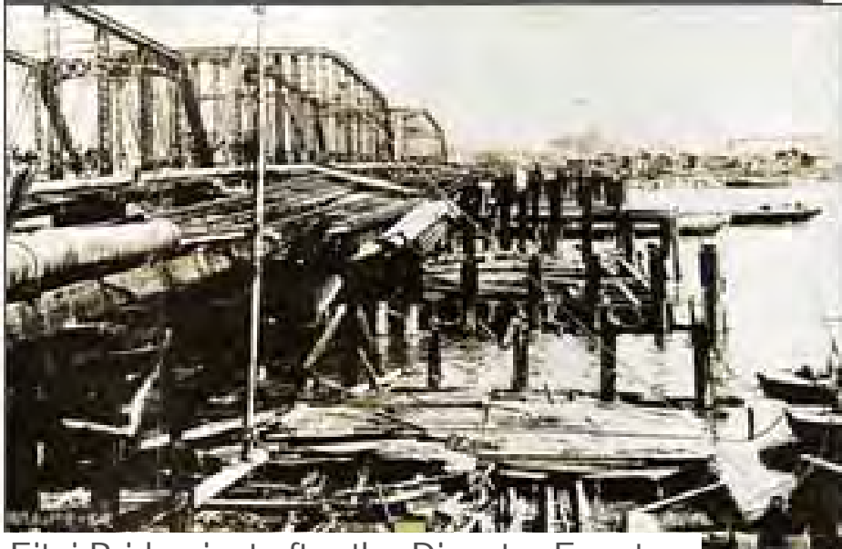
Eitai Bridge just after the Disaster Event
