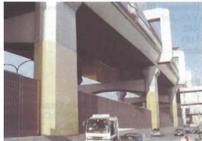
Figure 8 Strengthening for bridge piers
