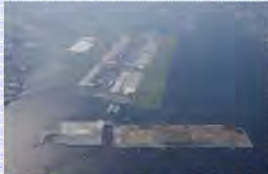
Re-expansion and internationalization of Haneda Airport (Photo courtesy of Haneda Airport Runway D Extension JV)
