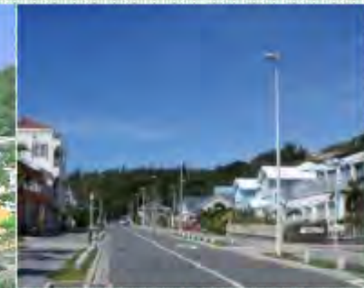
Underground installation of electricity cables (Ogasawara)
