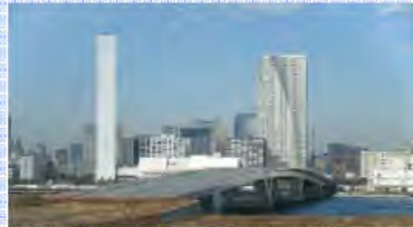
Toyosu-Ohashi Bridge on arterial ring route No. 2
