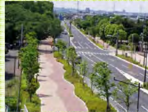
Creating expanded green space integrated with roads (Fuchu Tokorozawa Route)
