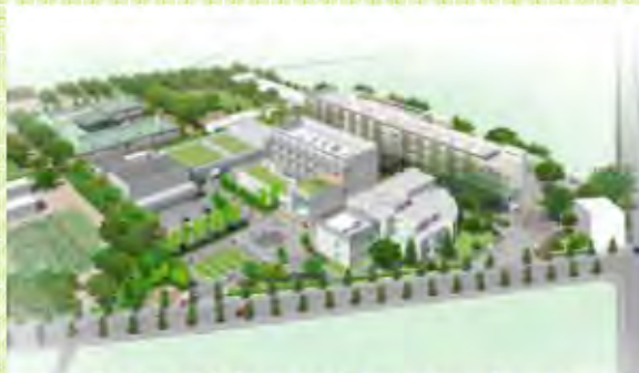
Industrial overall support base (Akishima City)
