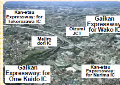
Gaikan Expressway Oizumi Junction Source: MLIT
