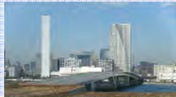
Toyosu-Ohashi Bridge on arterial ring route No. 2
