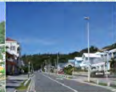
Underground installation of electricity cables (Ogasawara)
