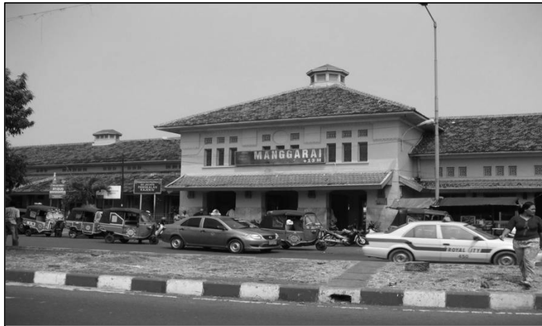
Existing conditions at Manggarai Station
