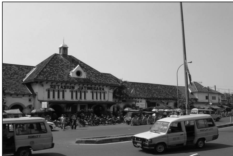
Existing conditions at Jatinegara Station
