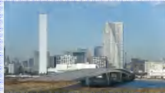
Toyosu-Ohashi Bridge or arterial ring route No. 2 (under construction)
