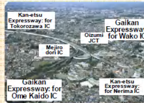
Gaikan Expressway Oizumi Junction
