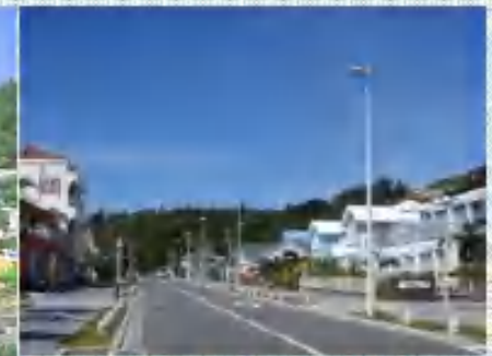
Underground installation of electricity cables (Ogasawara)
