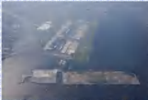
Re-expansion and internationalization of Haneda Airport (Photo courtesy of Haneda Airport Runway D Extension JV)
