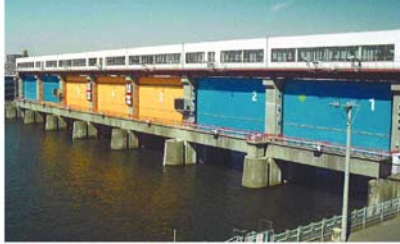
Sluice gate/ Drainage pumping station (photo: Imai sluice gate)
