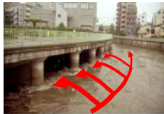
Inflow conditions at the Kanda River intake facility
