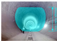
Inflow reached 90% of storage capacity (240,000m 3 )
