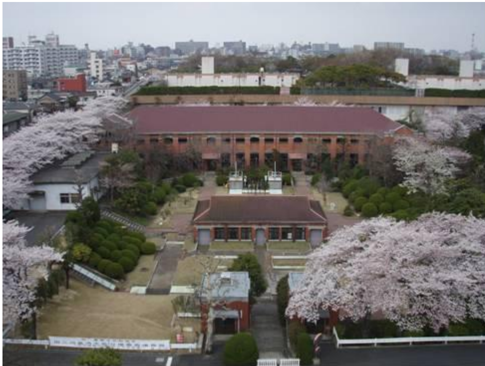
Pumping station in the old Mikawashima wastewater treatment plant (Important national cultural asset)
