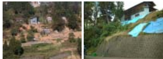
Damages by the Niigata Chuetsu Earthquake
