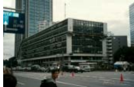
Damages by the Great Hanshin-Awaji Earthquake
