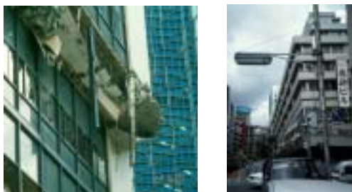
Damages by the Great Hanshin-Awaji Earthquake
