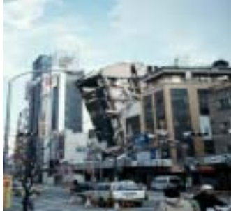
Damages by the Great Hanshin-Awaji Earthquake
