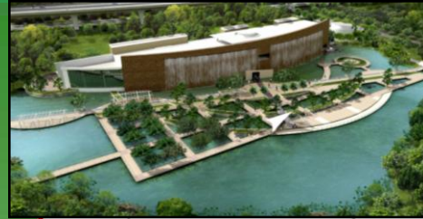
Bang Sue (Under construction)
