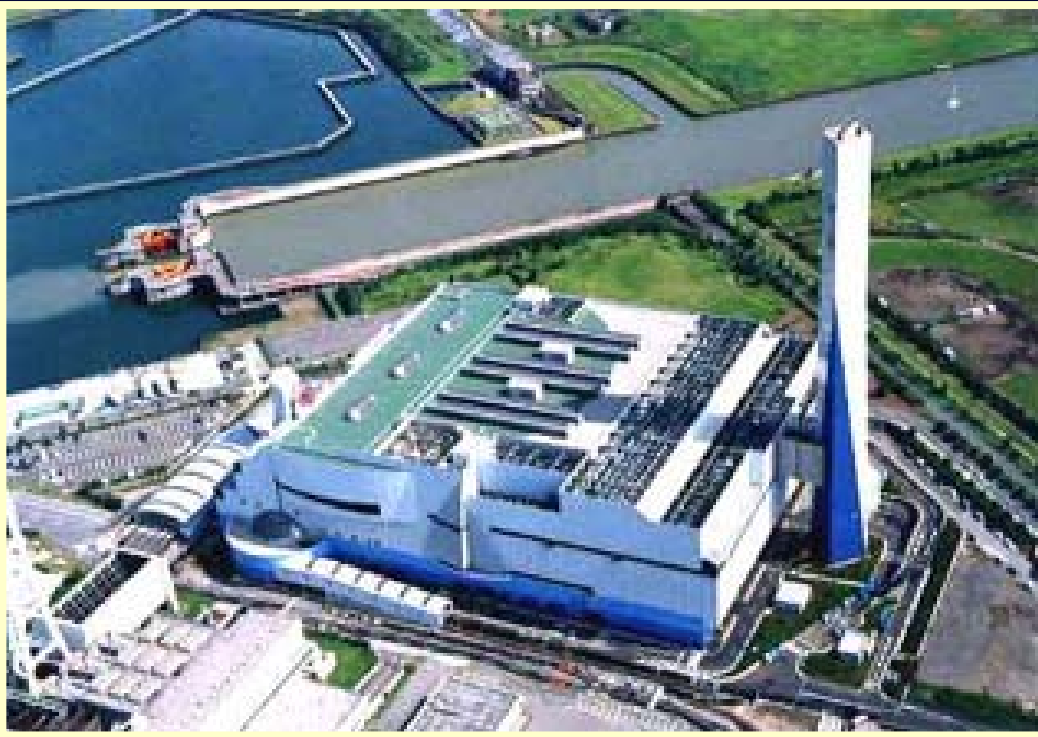
Shin-kouto incineration plant (capacity:1,800t/d) (power generation capacity :50,000kW)
