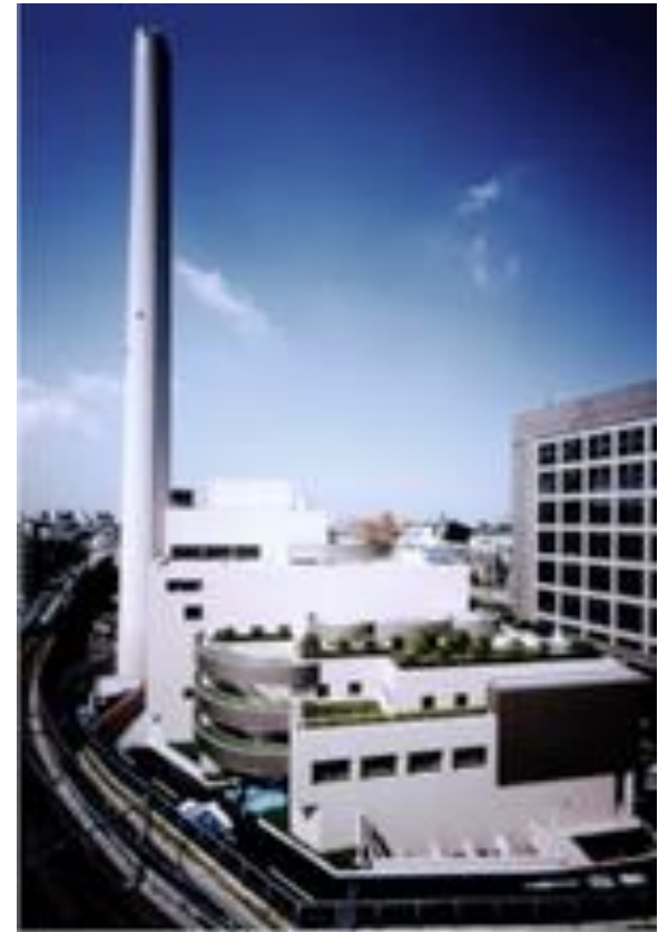
Shibuya Incineration Plant
