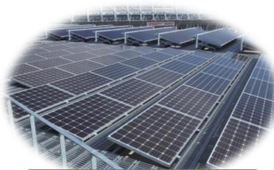
Preparations for power and communications outages, etc.
